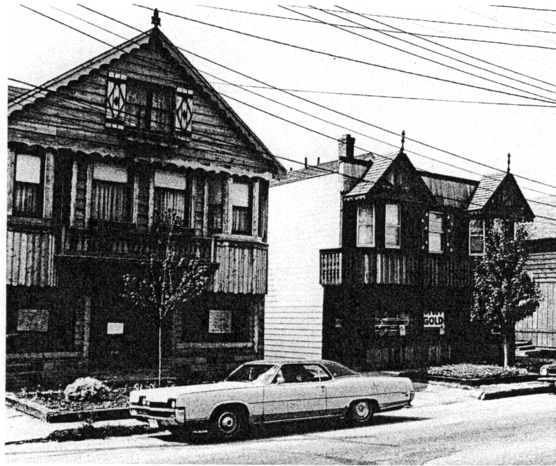
The Slavic Village renovation on Fleet Avenue.
