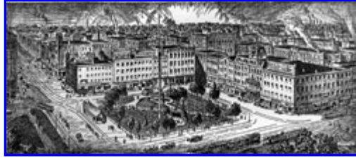
The southwest quadrangle as it looked prior to the station improvement.
